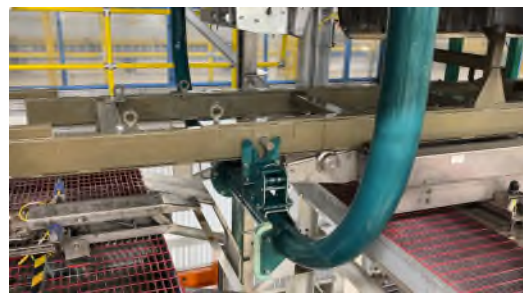
Skid transfer from pendul to outlet table
