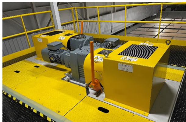
▲ Upper Caterpillar Drive Assembly – Main and Standby Drive Units
