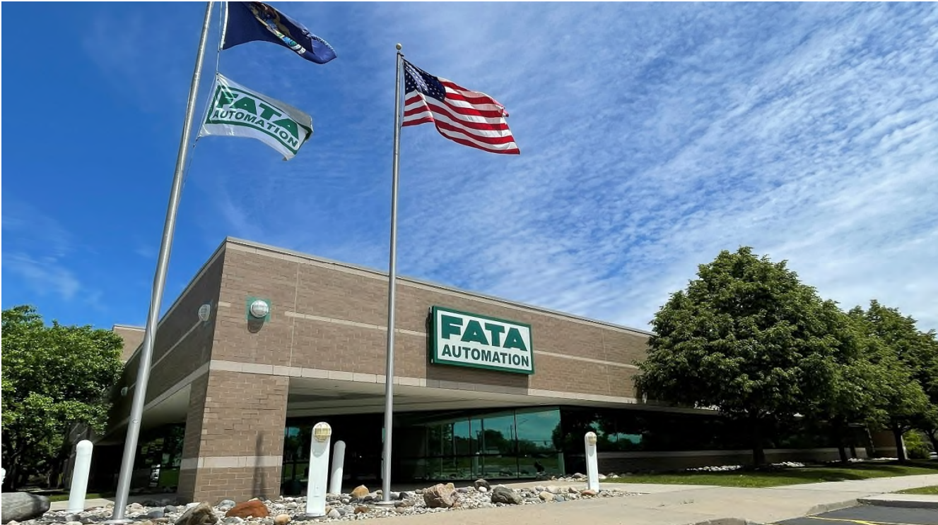
▲ FATA Automation Headquarters, Auburn Hills, MI
