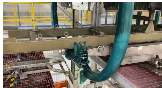
▲ Skid transfer from Pendul to outlet table.
